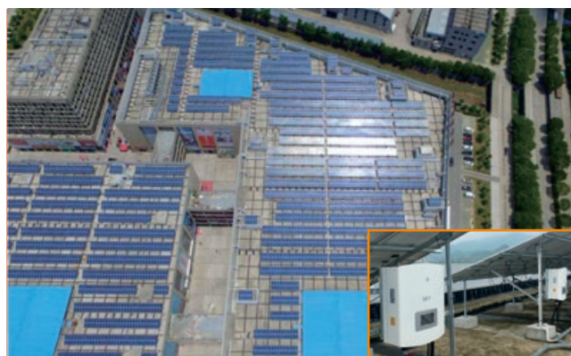
Ninghai AB hall, modern home plaza 1.53MW
