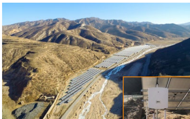
Shanxi Yizhou Jingle poverty alleviation PV Plant 36.3MW
