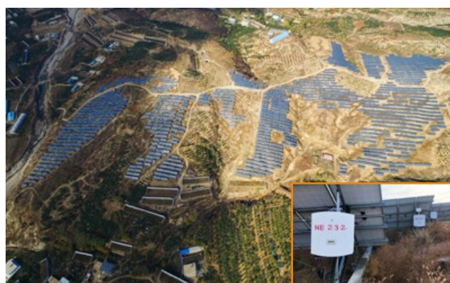
Liaoning Jiuzhai Gaizhou PV plant 20MW
