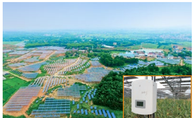
Quzhou Qinghu Agricultural-photovoltaic hybrid PV plant 20MW
