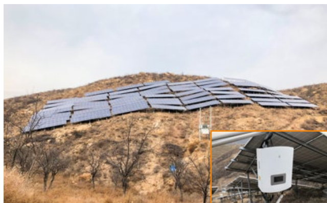
Hebei Baoding Fuping poverty alleviation PV Plant 6.6MW
