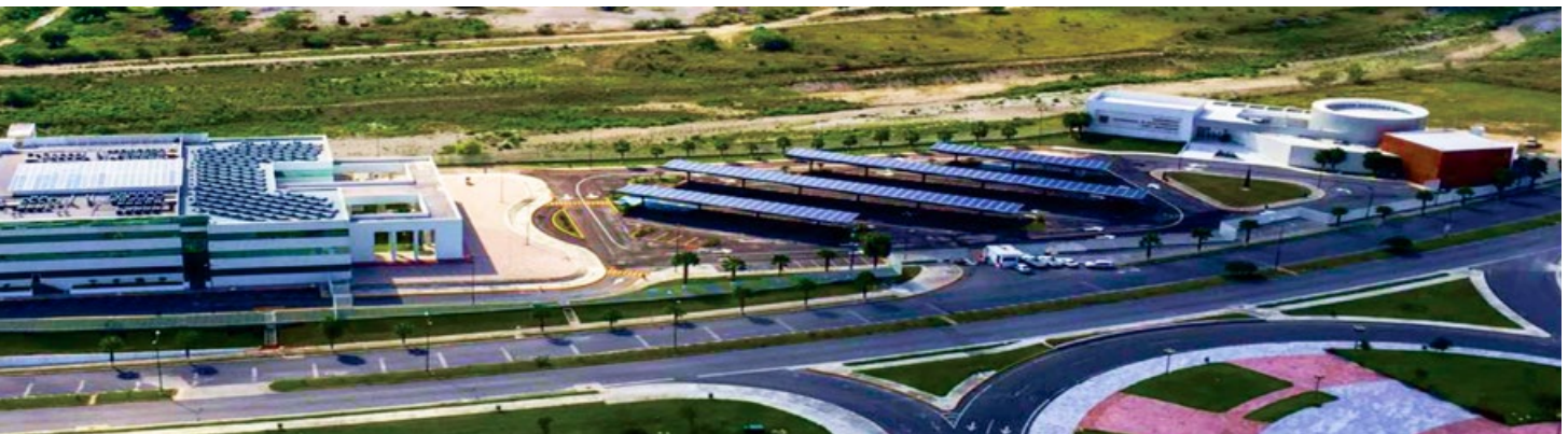
Mexico-Tamaulipas Carport, Mexico 5MW
