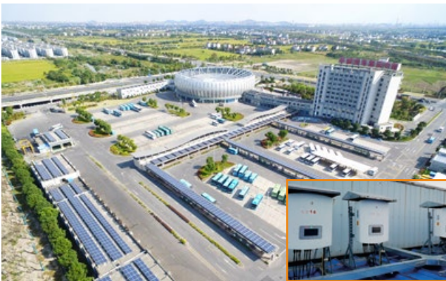
Zhejiang PINGHU Bus Station 472kW
