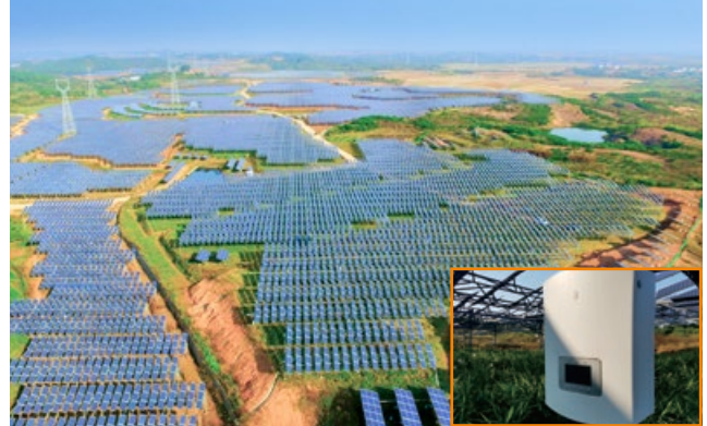
Zhejiang Hangbu Agricultural-photovoltaic hybrid PV plant 30MW
