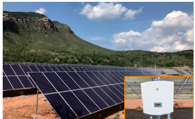
Shanxi Xiyang poverty alleviation PV Plant 7.2MW
