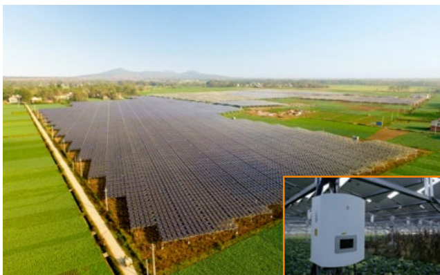
Hubei Guanyin Agricultural-photovoltaic hybrid PV plant 20MW
